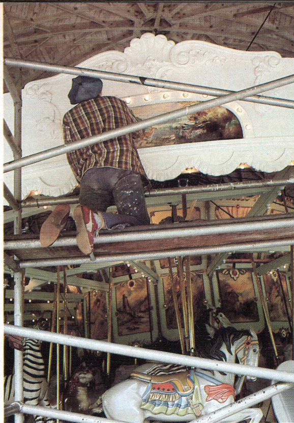
Part of the carousel restoration involved cleaning and revarnishing the painted panels on the outside rounding board.
